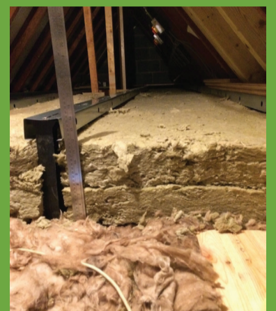
Insulate your loft – at least 25cm of insulation.
